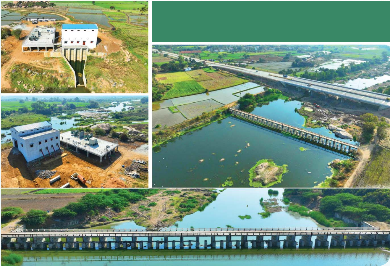
Ground Water Recharging Hirehalla Project with Fresh Water from Tungabhadra River 4 Tanks & 9 Barrages with 26.9ncft
