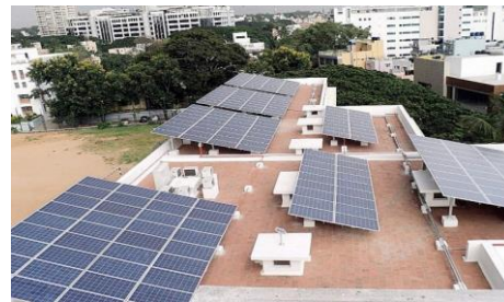
Installed Solar Panels at Surangi Unit, reducing 80 MT carbon emissions per month
