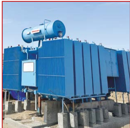
Inverter Duty Transformers (IDT) & Wind Turbine Generator Transformers for Renewable Energy
