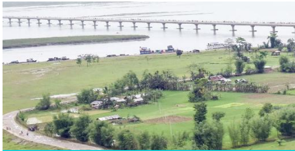
4 Lane Flyover at Mission Chairali, Tezpur, Assam
