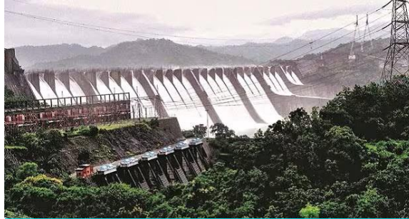
Lower Subansiri Hydro-electric Project, Arunachal Pradesh
