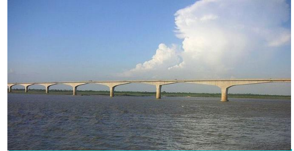
2 Lane Bridge over river Brahmaputra, Assam
