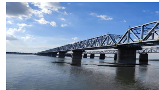
Steel bridge over river Ganga, Uttar Pradesh
