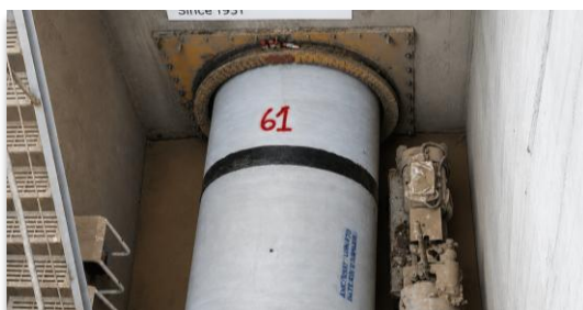
Ahmedabad Micro Tunnelling, Gujarat
