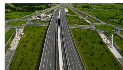
Ganga Expressway, Uttar Pradesh
