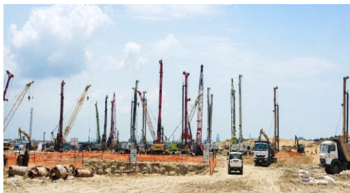
Piling work, Odisha
