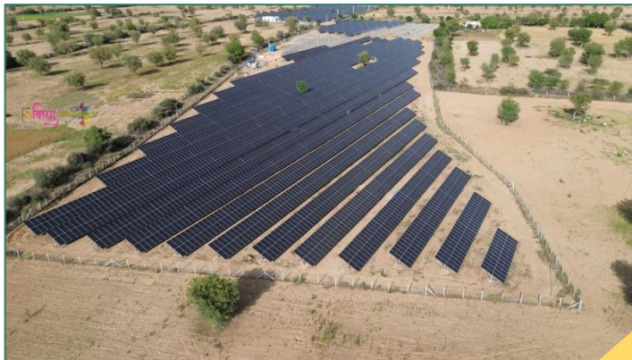
7.52 MWp Capacity Solar On Grid project commissioned under PM KUSUM C yojana.
