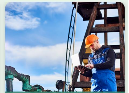
WATER UTILITY SHIFTING WORK
