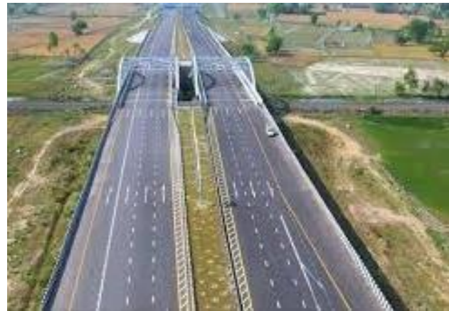
Up to 33KV Electrical Utility Shifting, Aligarh-Kanpur Highway
