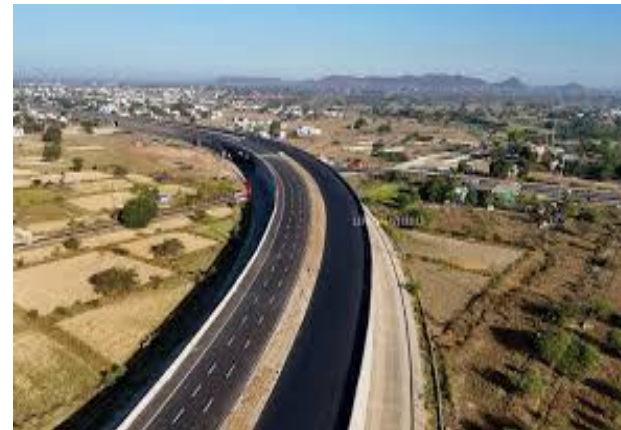
Electrical Utility Shifting Work upto 33KV in Maharashtra
