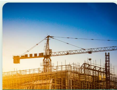
INTERIOR & CIVIL WORK
