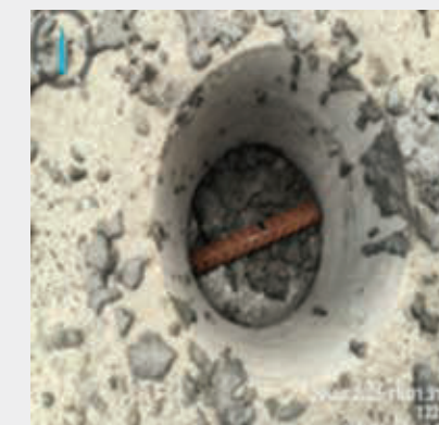
Treatment of cracks through epoxy resin injection
