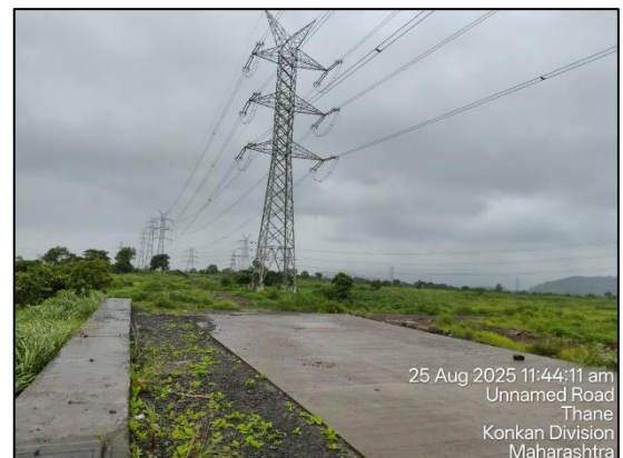
Access road to the subject property
