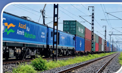
Double Stack Container Train on Dedicated Freight Corridor
