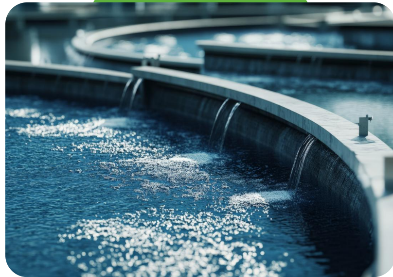
Shotts Waste Water Treatment Works, Glasgow UK
