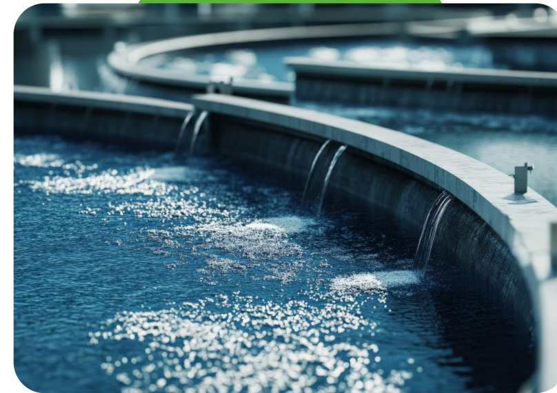
Shotts Waste Water Treatment Works, Glasgow UK
