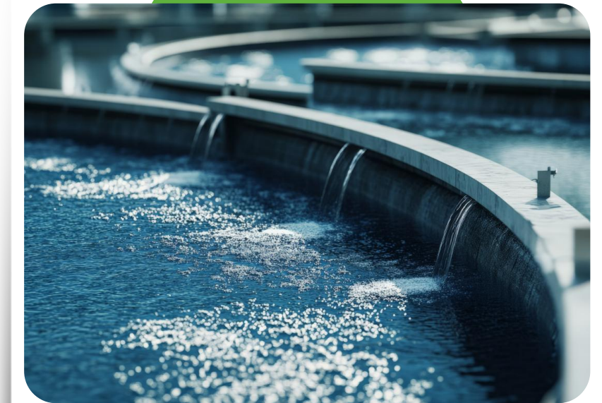
Shotts Waste Water Treatment Works, Glasgow UK
