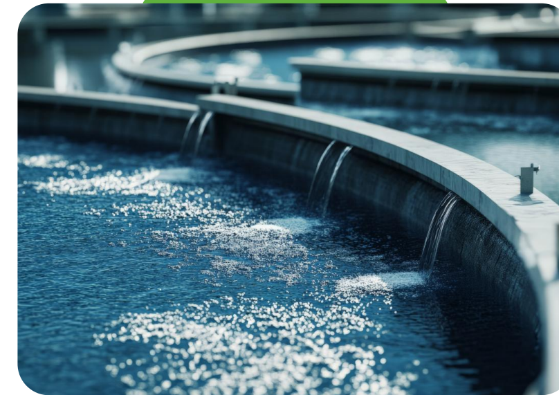
Shotts Waste Water Treatment Works, Glasgow UK
