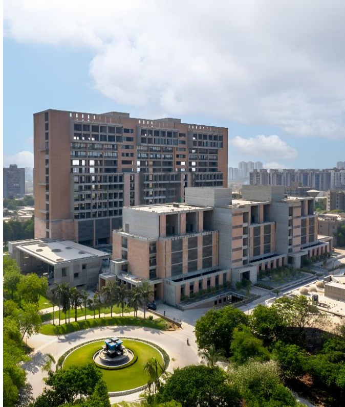
Nirma University – Old Building
