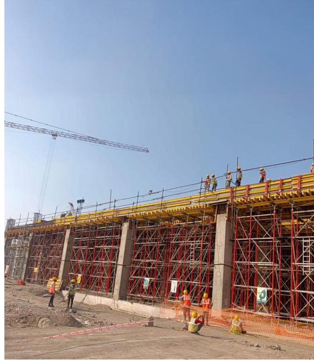
Equipment name : Peri Up MI System for Beam Bottom Country of origin : Germany Amount invested : ₹18.8 crores
