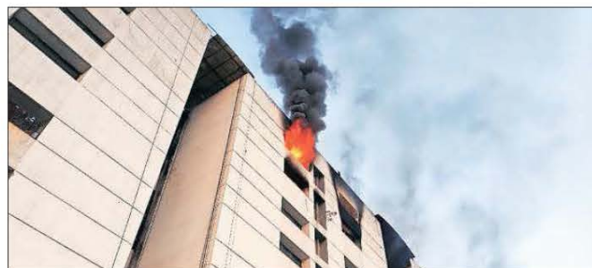
The fire broke out in a six-storey building. EXPRESS
