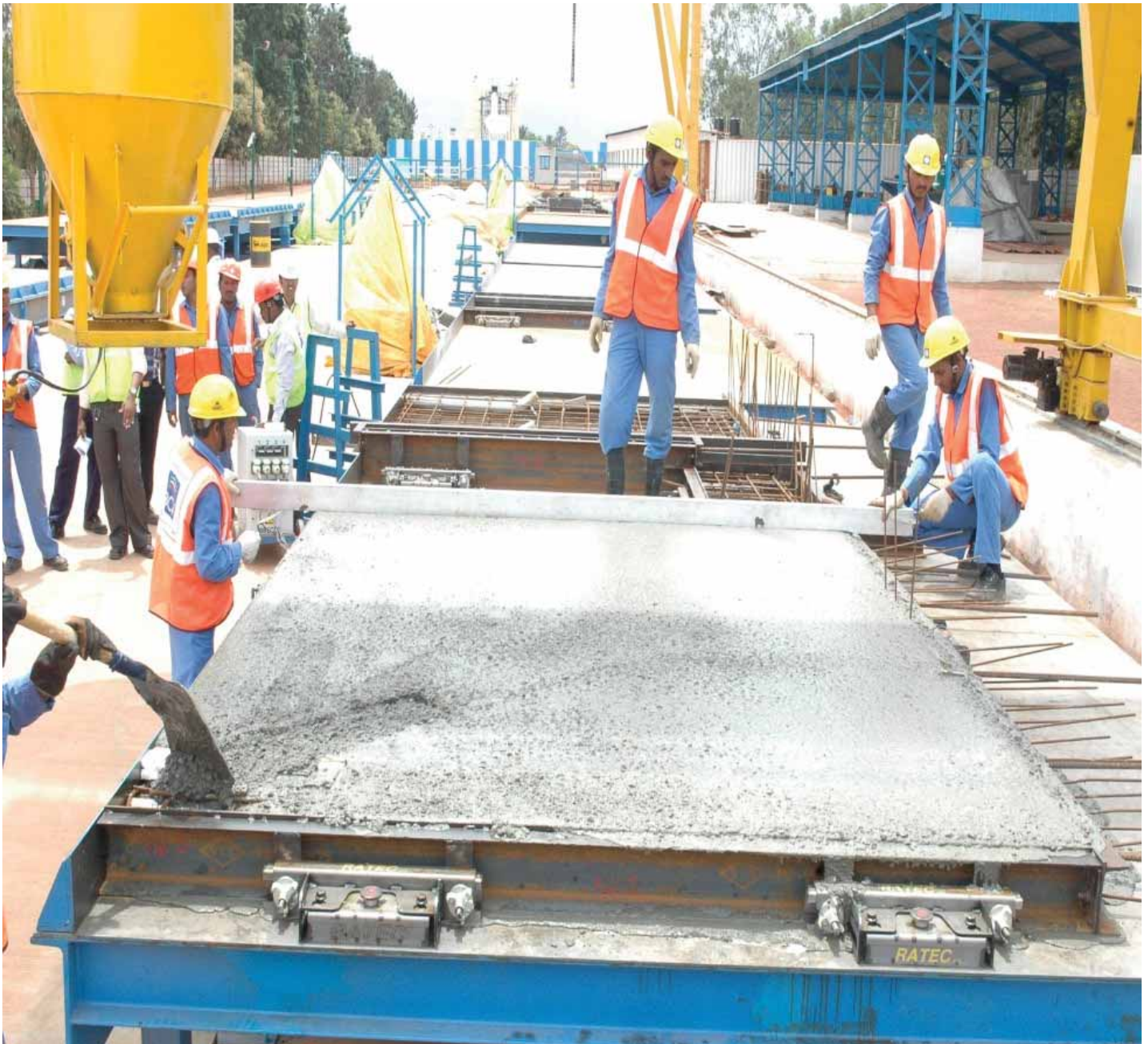
Shot at Location- Precast Plant
