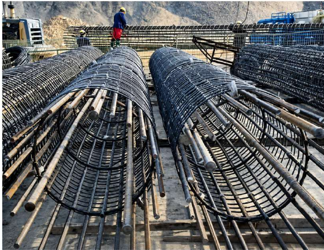
TMT bore piling
