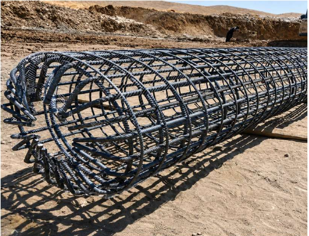
Ready built steel
