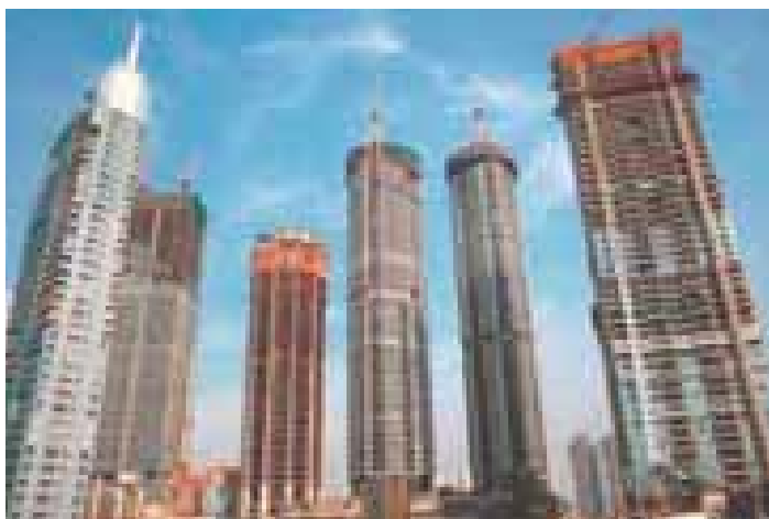
HVAC services for Omkar Realtors & Developers, Mumbai
