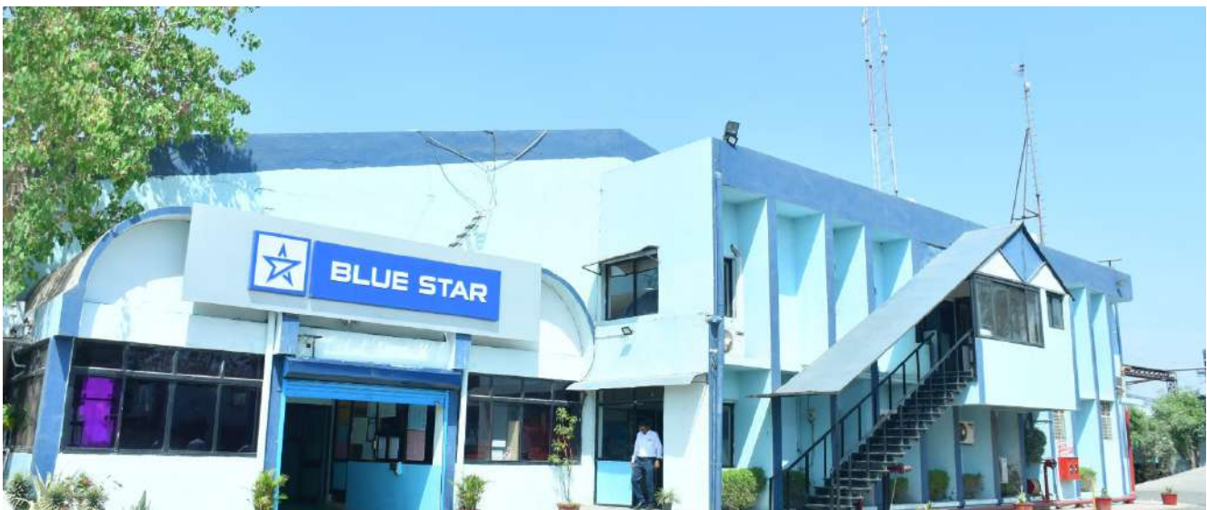
Blue Star's manufacturing facility at Ahmedabad
