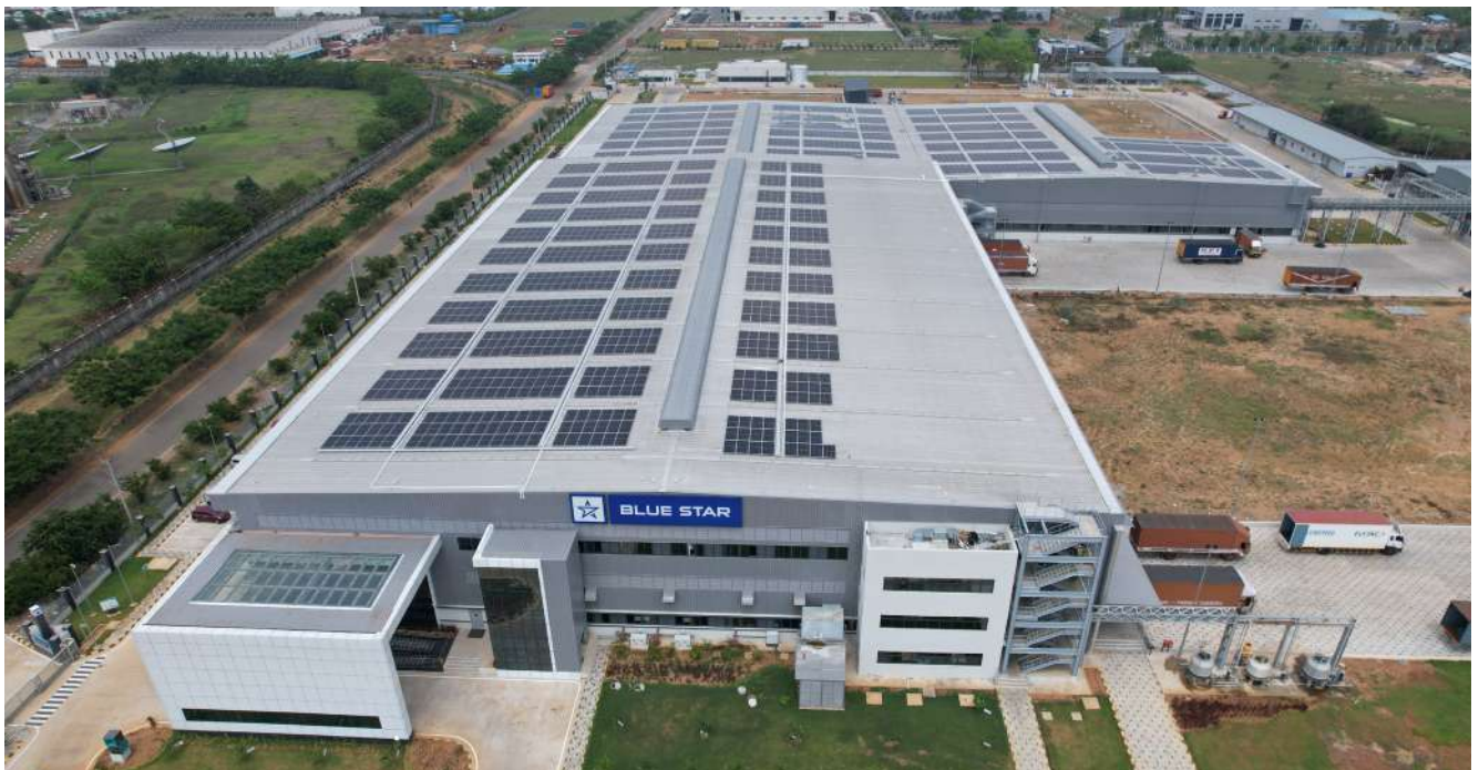
Blue Star Climatech Limited's state-of-the-art Sri City Plant
