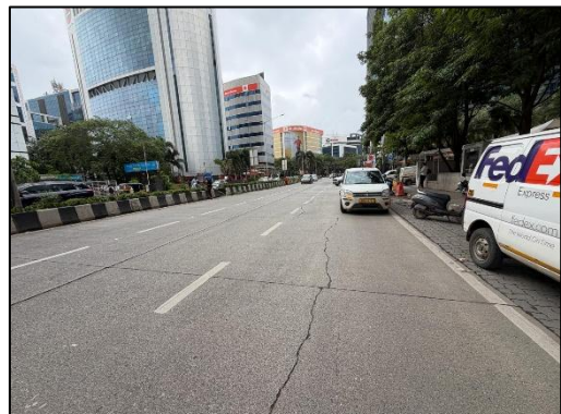
View of the access road (Lane 3 Road)
