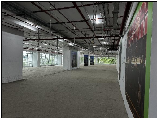
View of the Vacant Area on Floor 2
