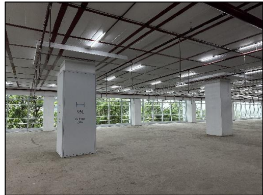
View of the Vacant Area on Floor 2
