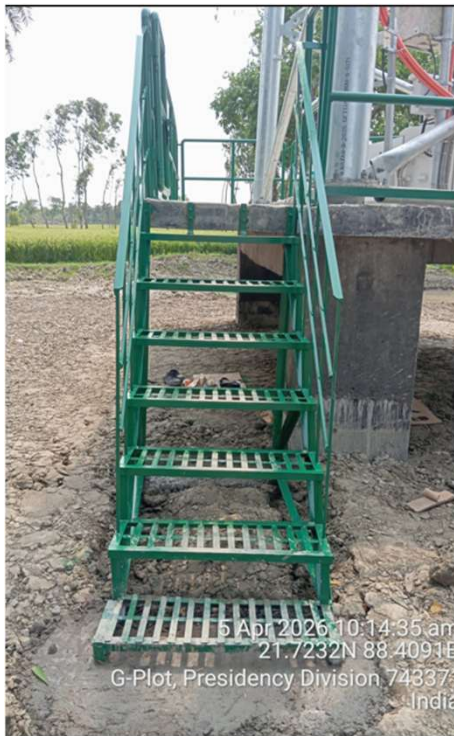
Elevated Flood Mitigation Foundation
