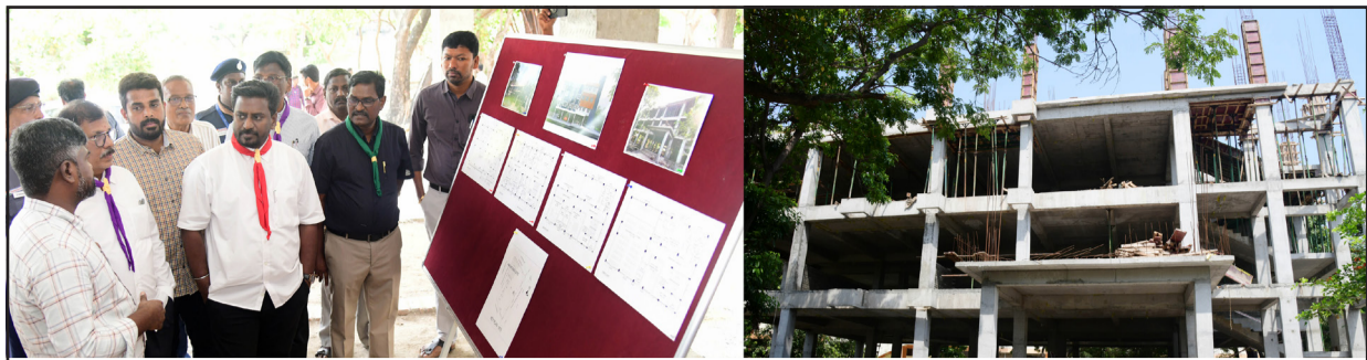
School Education, Tamil Development, Information and Publicity Minister Raj Mohan inspected the construction works of the new Bharat Scouts and Guides State Headquarters building being constructed at a cost of Rs.8.93 crore in Kamarajar Salai, Chennai. School Education Director S. Kannappan, Elementary Education Director P.A. Naresh, Assistant Executive Engineer Senthil Raj, Assistant Engineer Tamilarasi, and senior government officials accompanied him during the inspection.
