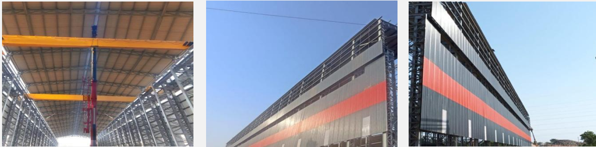
Note : The above are on ground images of the greenfield manufacturing campus
