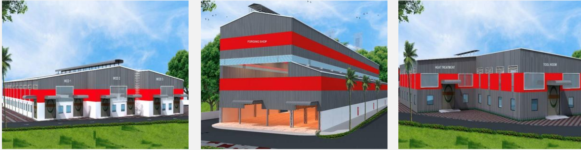
Note: The above is a 3D illustration of the greenfield manufacturing campus
