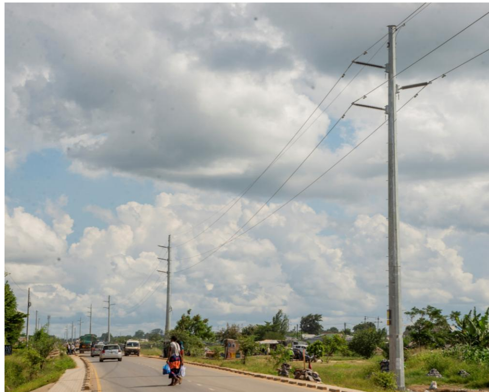
Construction of 132kV Single Circuit Transmission Line from Coventry – Waterworks, Coventry – Jimmy – Chawama for ZESCO in Lusaka
