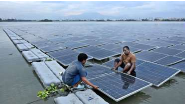
TARIFF ADJUSTMENT. The accelerated build-out was driven by the phased removal of waivers for transmission charges
