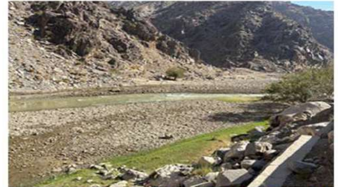
Photographs 1: Downstream view of the proposed diversion structure of Surobi-2 project site.
