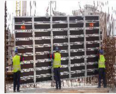
MIVAN construction technology
