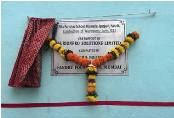
Construction of Toilet, Rajwada School
