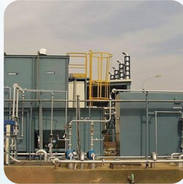
Prefabricated Sewage Treatment Plant
