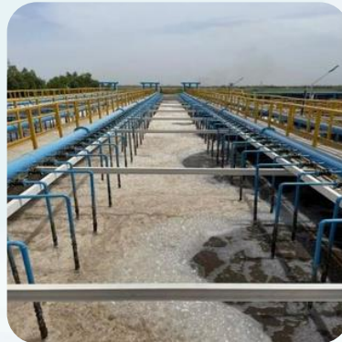
STP Based On Membrane Bioreactor
