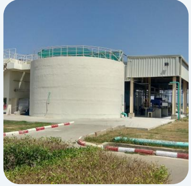
Pre-treatment Clarification & Pumping System
