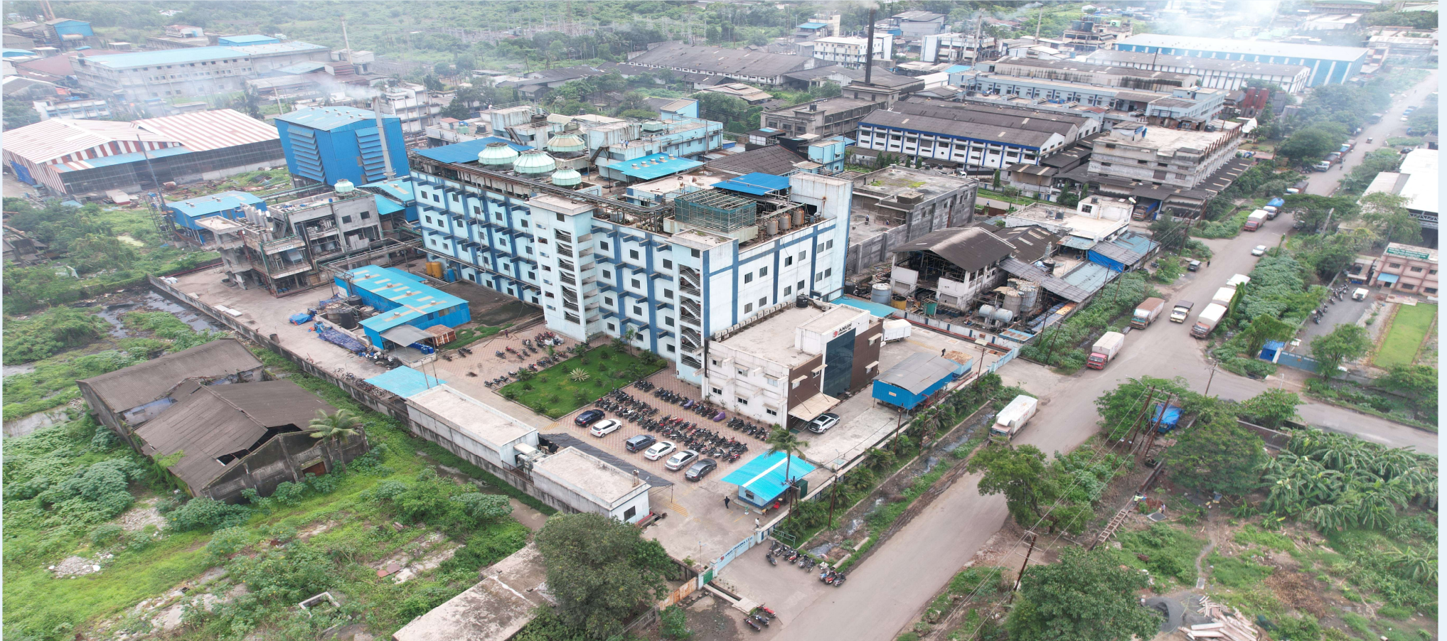
Aerial view of the Tarapur manufacturing complex - 9 API blocks and 2 intermediate blocks.
