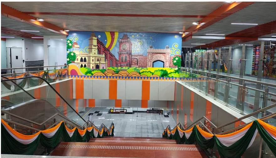
Kanpur Central Metro Station built by Afcons
