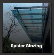
The term "spider" refers to the specialized fittings or point-fix connectors that hold and support glass panels. Spider Glazing is the ideal solution for creating large, open entrances in commercial or residential buildings. Most modern exterior design concepts rely on this structural glazing system to achieve expansive, seamless class facades.
