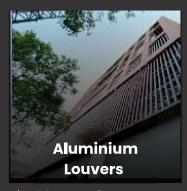
Aluminium louvers are architectural elements designed to enhance building aesthetics while providing ventilation and natural light control. Made from lightweight, durable aluminum, these horizontal or vertical slats allow airflow and light to pass through while offering privacy and protection from the elements
