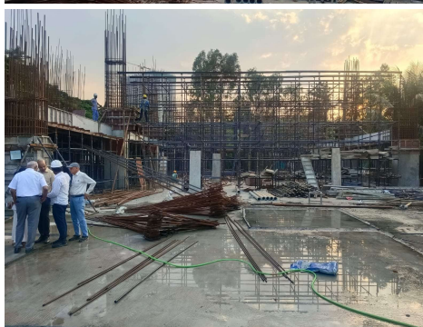
Construction in progress at the Bhosari site
