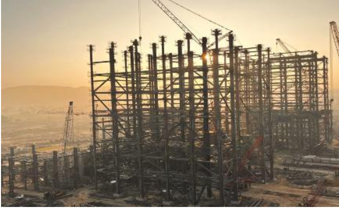
Unit #3 Electrostatic Precipitator Hopper erection work progress
