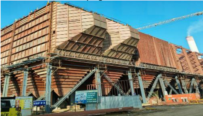
Unit #3 Electrostatic Precipitator Hopper erection work progress
