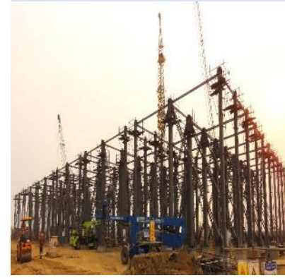
Unit #3 - Electrostatic Precipitator
