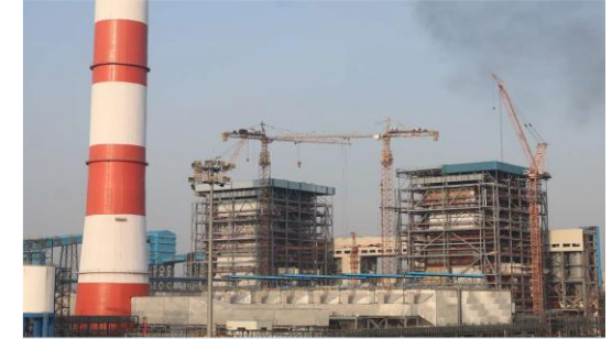
High Pressure Feed Water Heater Insulation
