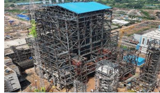
Boiler Column Structure Erection
