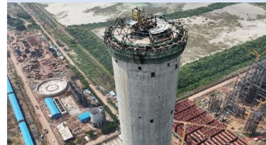
Chimney Wind Shield Completed
