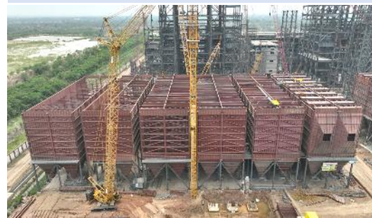
Junction Tower Structure erection
