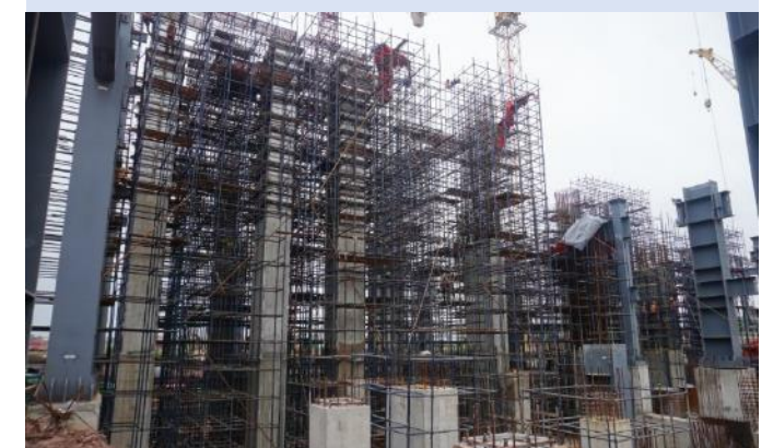
Unit #2 Turbine Generator Deck Column Casting
