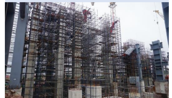
Unit #2 Turbine Generator Deck Column Casting
