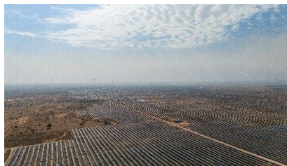
2,140 MW at Jaisalmer, Rajasthan
