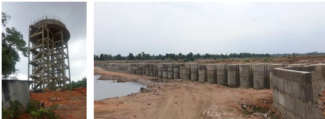
Current Images of the Project Site
