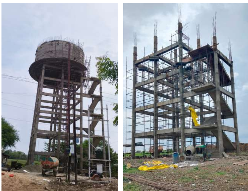
Current Images of the Project Site
