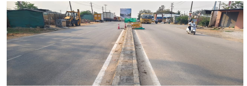
Phase III external road construction underway at Nelamangala
