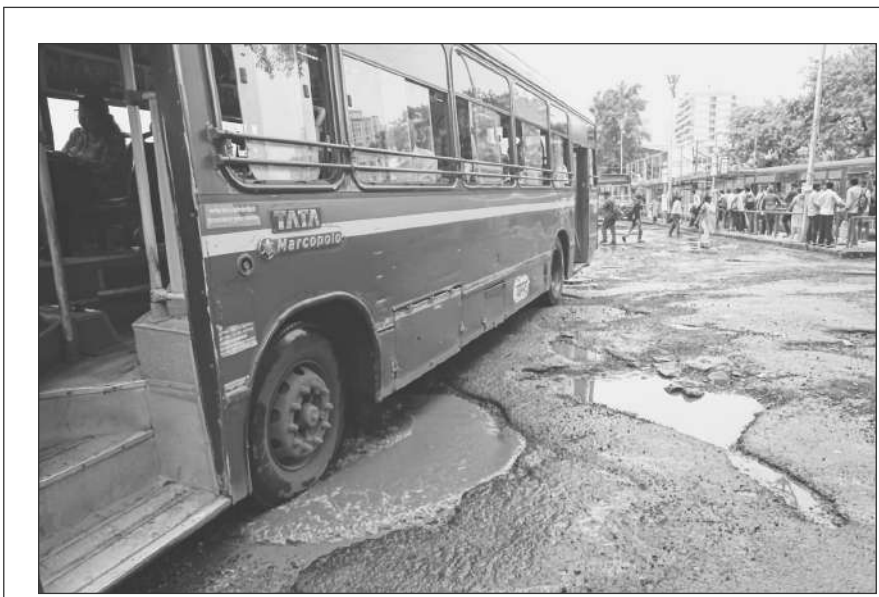
Road woes Huge potholes at the Goregaon BEST Bus Depot pose safety concerns for buses and daily commuters. — Vijay Gohil
