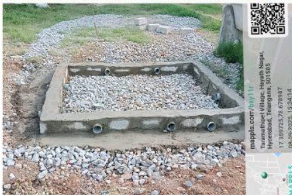
Rainwater Harvesting Pit at ZPHS Tharamathipet School, Rangareddy District. Successfully Completed. 08.09.2025
