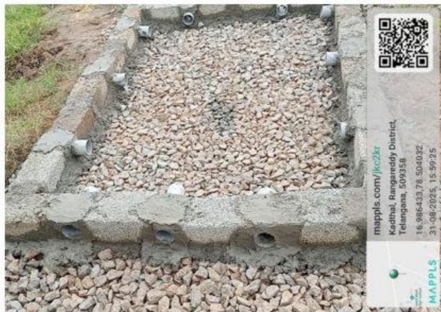
Water Harvesting pit 31.08.2025
