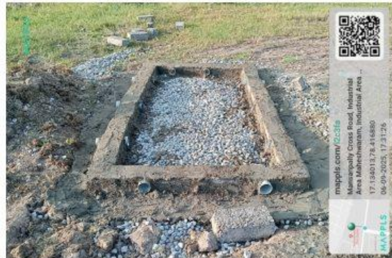
Water harvesting pit completed 06.09.2025.
