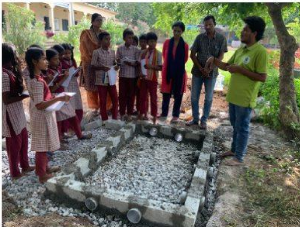
WaterHarvesting pit Demonstration @ZPHS Janagama 03.09.2025
