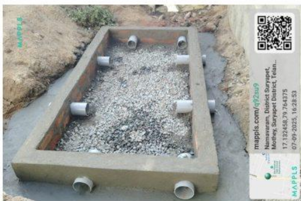
Water Harvesting Completed 07.09.2025.
