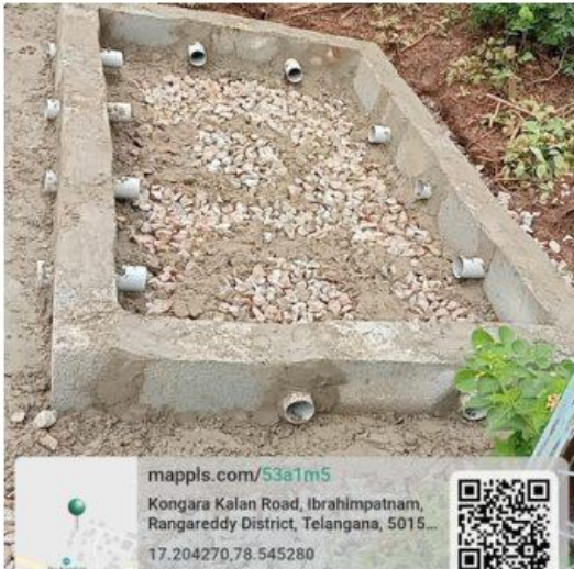
Water Harvesting Pit completed on 11.09.2025
