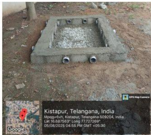
water harvesting pit completed narayana pet 05.08.2025
