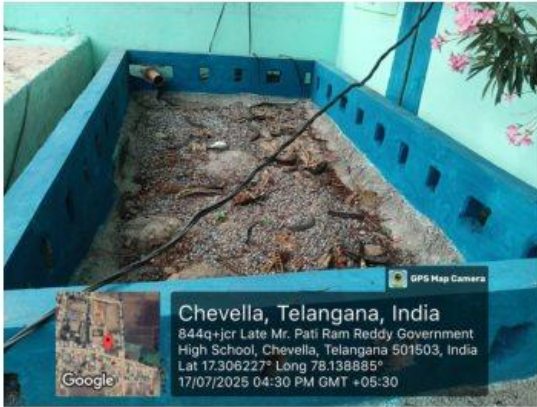
Rainwater Harvesting at PM Shri TGMS, Chevella, Rangareddy District."
