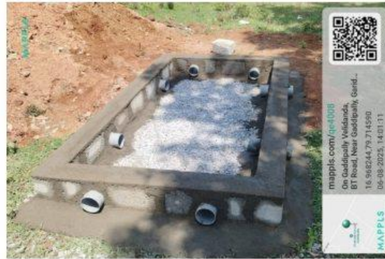
TGMS Gaddipalli, Suryapet District, work has commenced for the water harvesting pit and compost pit.
