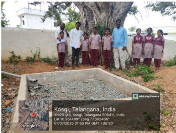
Rain Water Harvesting pit 07.07.2025
