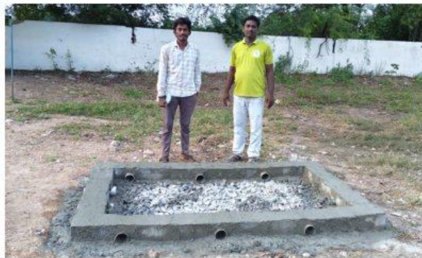
Water Harvesting Pit completed at ZPHS Narva, Narayanpet District. 05.08.2025.
