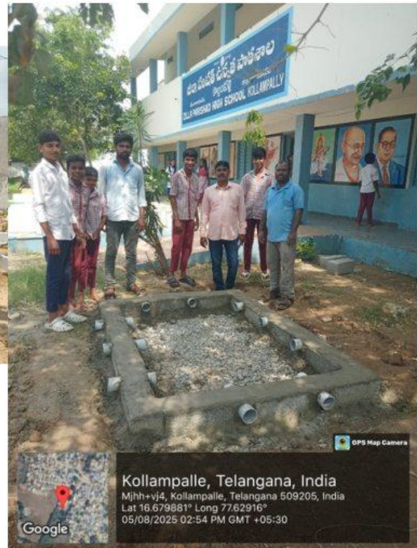
Water Harvesting Pit completed at ZPHS Kollampalle, 05.08.2025
