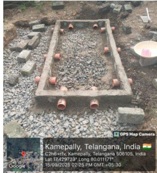
PM SHRI ZPHS KAMPALLY Rain water harvesting work done 15.09.2025
