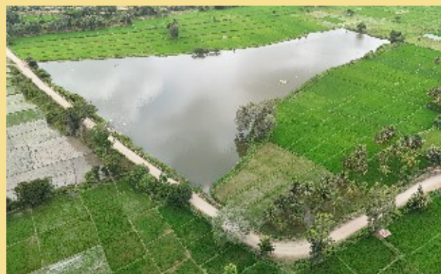
Tank Desiltation Work at Mavathuru Village
