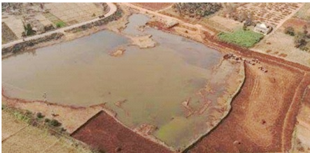
Area Treatment at Chitikyathanahalli Village
