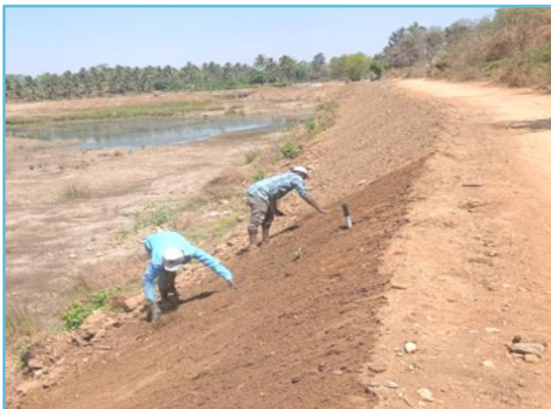
Lake Improvement works at Sheshagirihalli Lake
