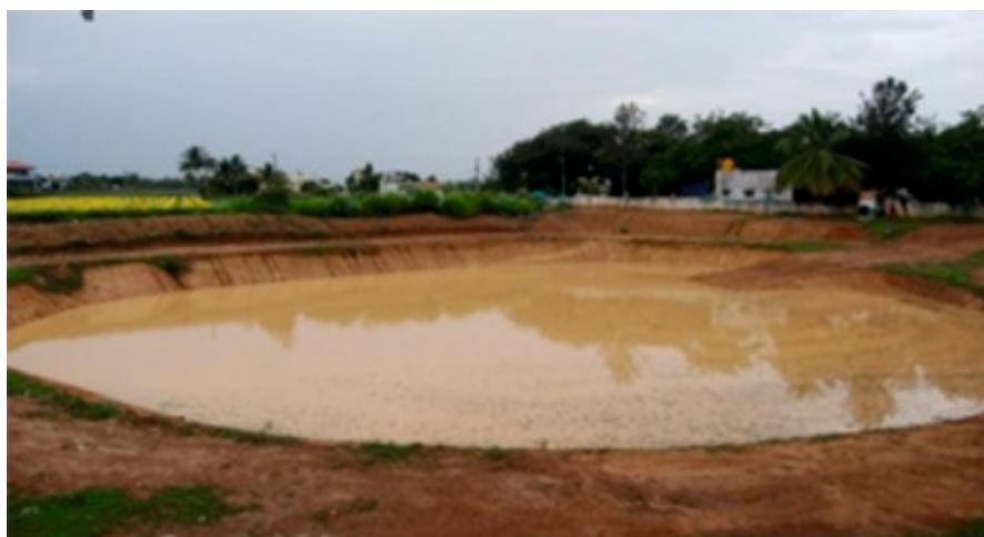
Pond Restoration Work at Shivanapura Village
