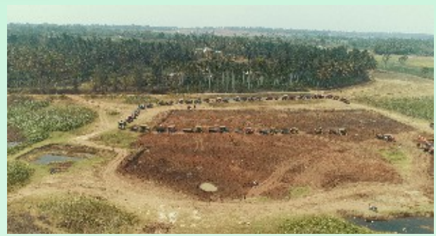
Tank Work at Chowdikatte Village
