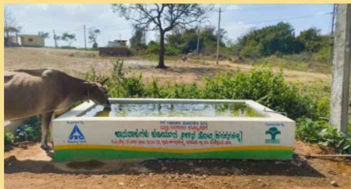
Cattle Trough Construction at Hagaranahalli Village
