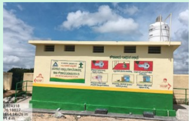
School Toilet Construction at GHS Banadahalli
