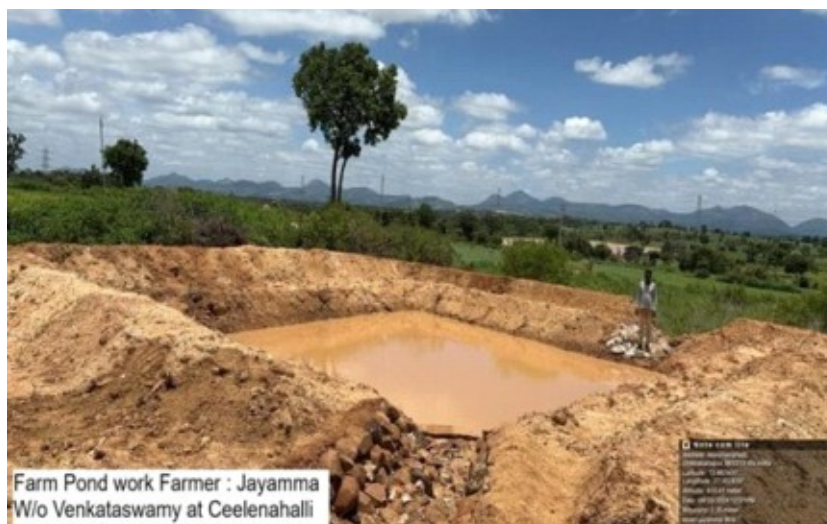
Farm Pond work at Chelenahalli
