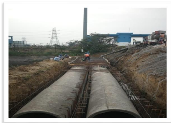
Modification to existing Run-Off Pits
