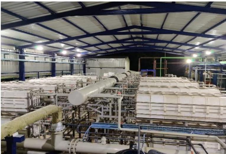
Waste heat evaporator plants are modular treatment systems using thermal energy to extract clean water from highly concentrated waste waters and reverse osmosis plant rejects.
