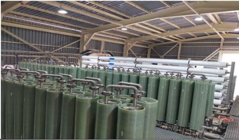
membrane systems help mitigate this by reducing the evaporator load, thereby decreasing steam consumption and lowering operating costs.
