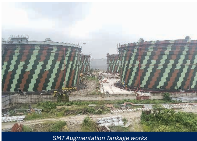
SMT Augmentation Tankage works
