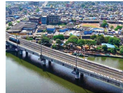
➤ Dedicated Freight Corridor
