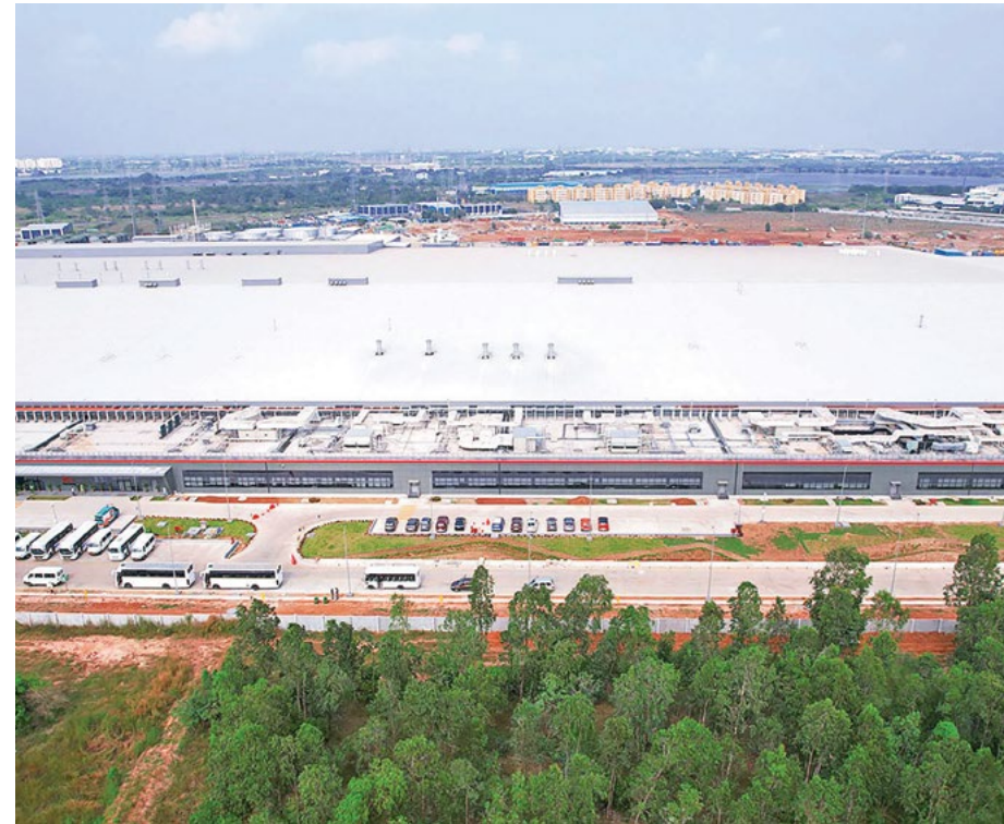
➤ Solar Factory for First Solar
