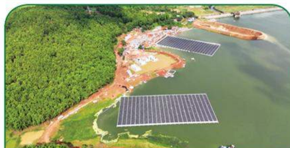
100 MW Floating Solar PV Power Plant at Getalsud Dam, Ranchi, Jharkhand
