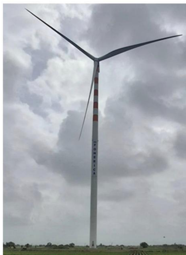
50 MW Wind Power Project, Devbhoomi Dwaraka, Gujarat under SECI Wind Tranche -XVI awarded to M/s Powerica Ltd
