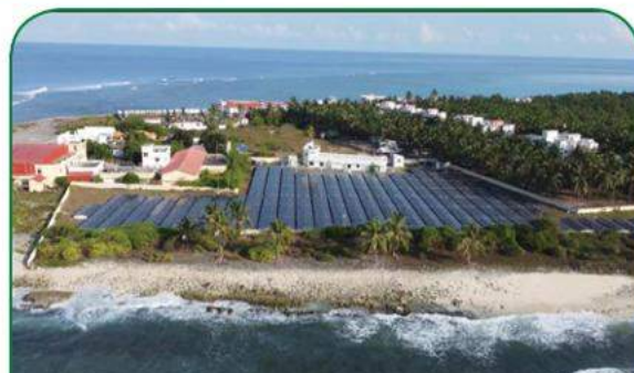
1.7 MW Solar PV Power Plant with 1.4 MWh BESS at Lakshadweep
