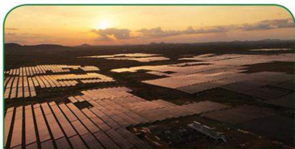
300 MW Solar PV Power Plant at Ramagiri, Andhra Pradesh
