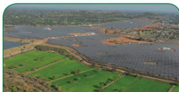
100 MW Solar PV Power Plant along with 40MW/120 MWh BESS at Rajnandgaon, Chhattisgarh
