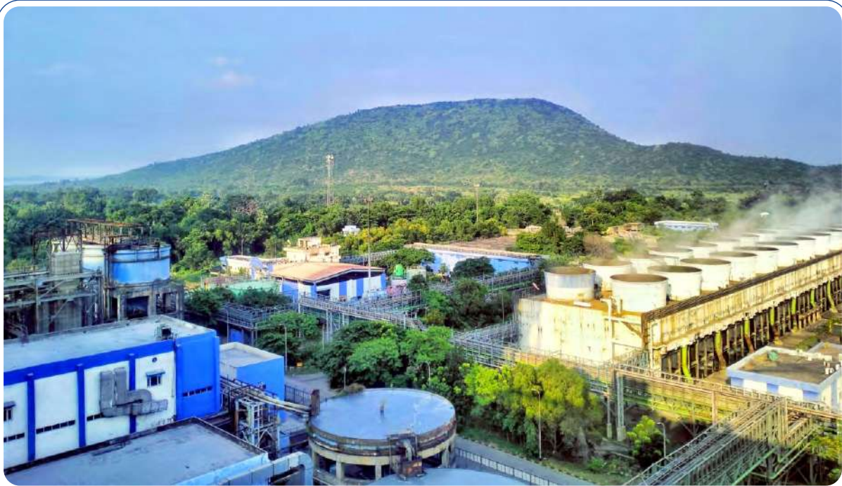
Birds eye view of the Balance of Plant Area and Cooling Towers
