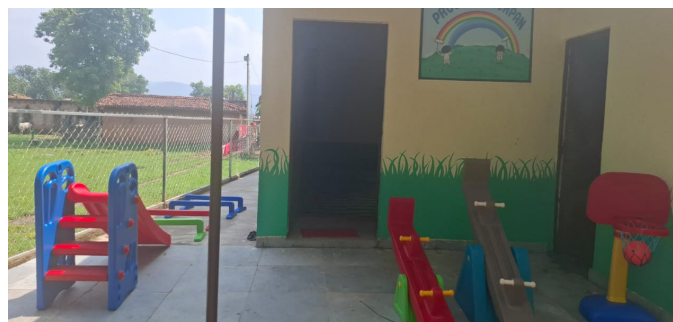
New Bachpan Centre at Harni (Turiya) village of Khaira block (Jamui)
